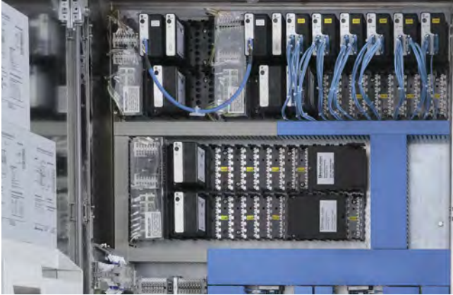
Figure 3 Stainless steel FB Remote I/O enclosure
