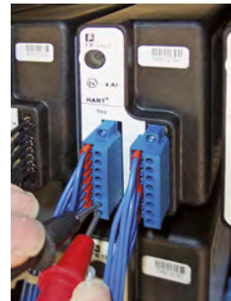
Figure 14 Applying the Handheld Communicator
