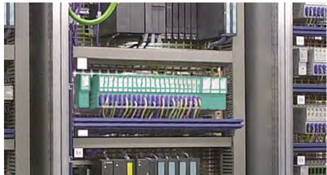
Figure 1 Control room installation
